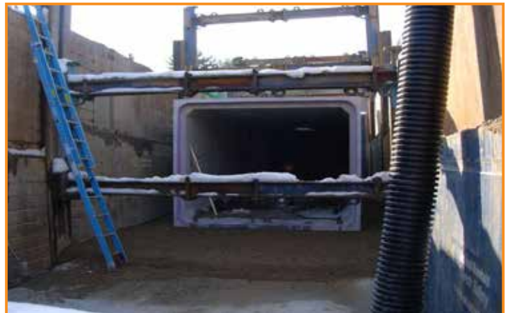
Linear system used for a large vault
